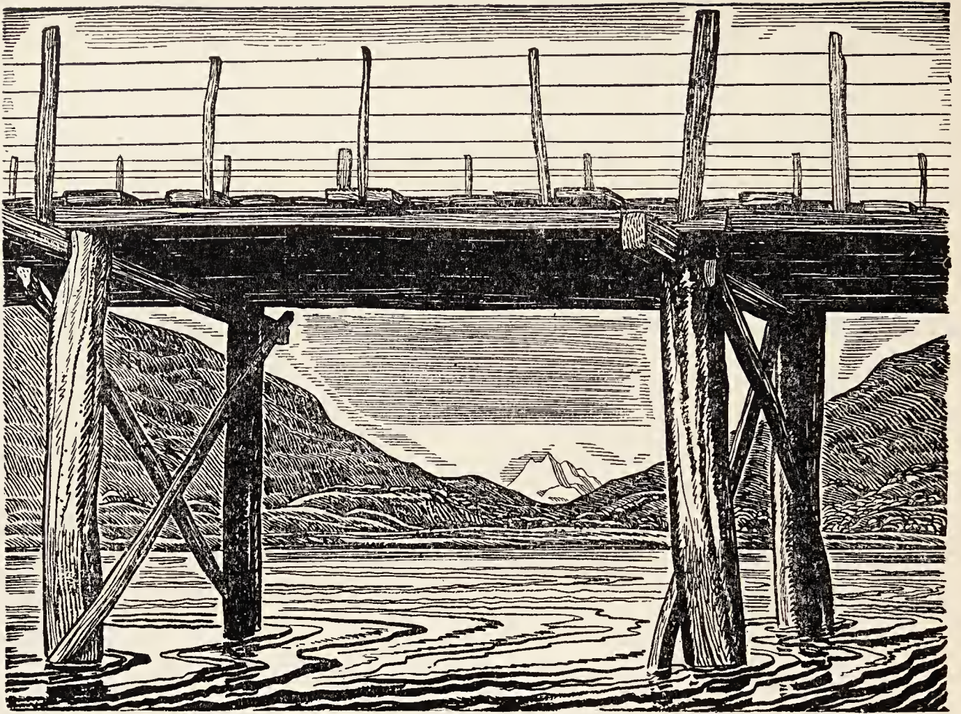
BRIDGE ACROSS AZAPARDO RIVER
